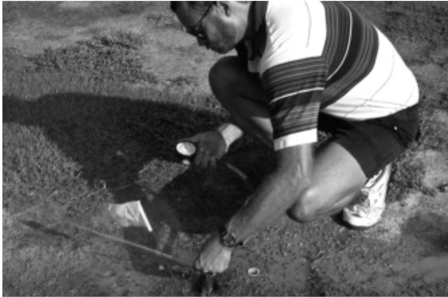
Check water pressure at each sprinkler and record pressure problems.
